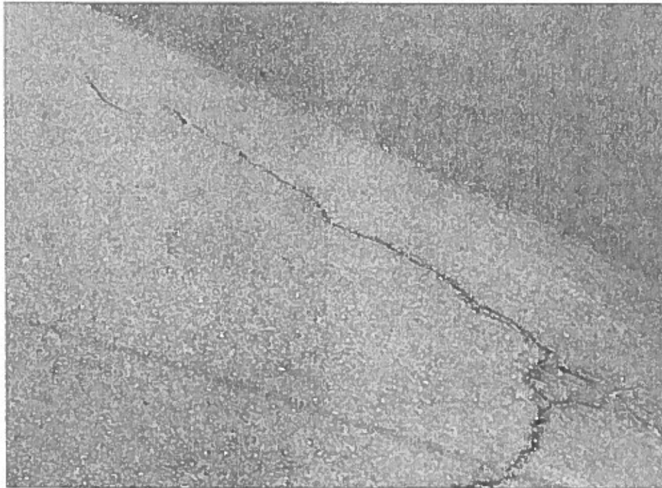
Figure 2: Medium cracking
