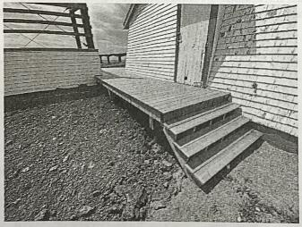
2. Steps were constructed with hinges to move with the ground. This is not acceptable as it is a public entrance for the deck. The steps need to be secured and solid at ground level below frost with continuous railing, with a 1' extension beyond the end. Treads are not wide enough (11" minimum). Steps to be reconstructed to be three 1x6 wide. Landing at deck to be extended to existing deck.
