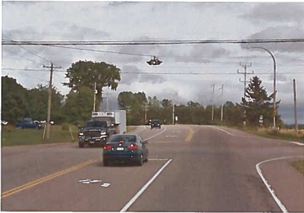
Figure 4 – Eastbound approach: Overhead flashing lights
